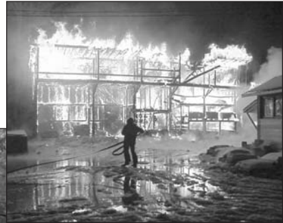
Figure 31- The Company survived a January 2002 fire that was started by youths
